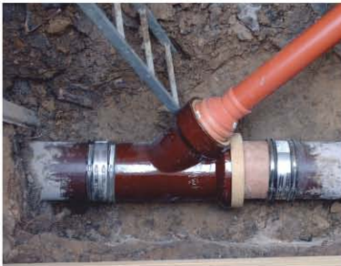
Reparatur in offener Baugrube
